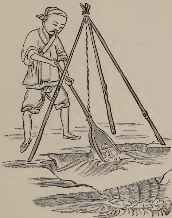
LIFTING WATER BY TRIPOD FRAME.
